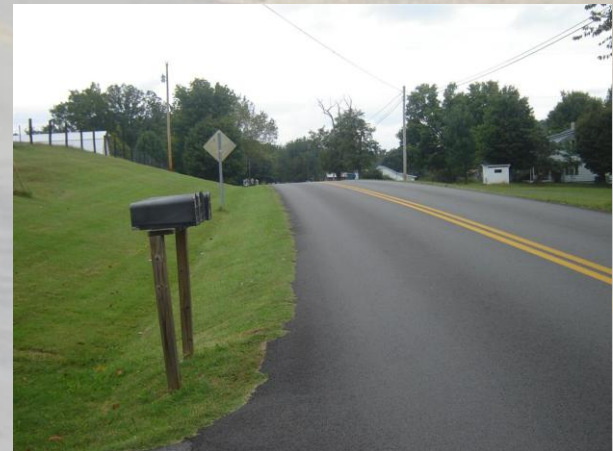
Substandard Vertical Curve
