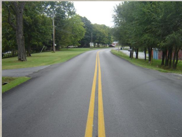
Substandard Horizontal Curve
