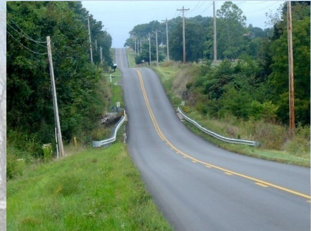
Existing Black Rock Creek Bridge
